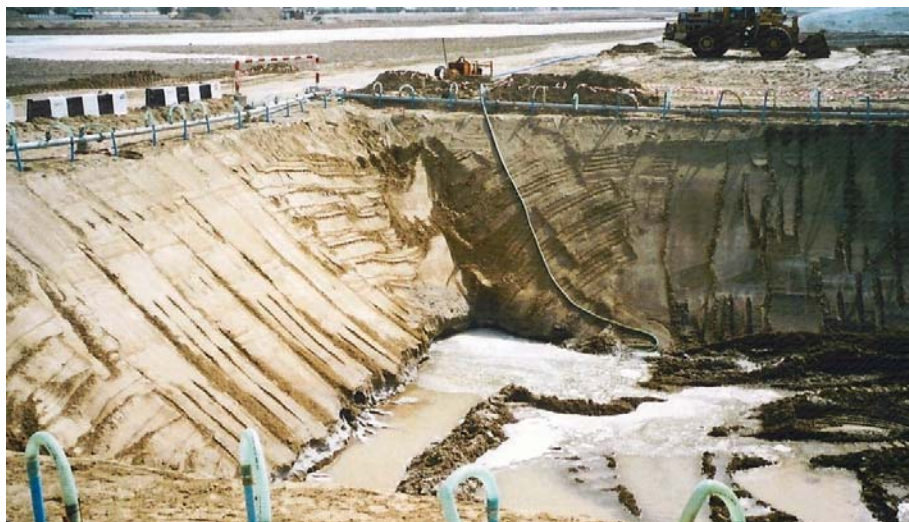
Fig 3. A temporary pit near the junction of the Aryam road with the main Abu Dhabi-Jebel Dhanna coast road. At least six metres of brown sand are exposed. It probably extends beneath the whole of Al Aryam. (The apparent cross-beds are actually digger markings).
